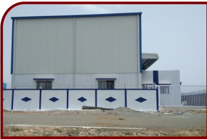
Fourtech Engineering Enterprises, Chakan
